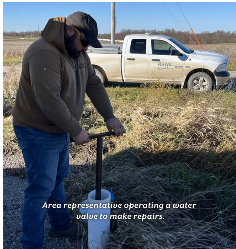
Area representative locating and marking a water main.
