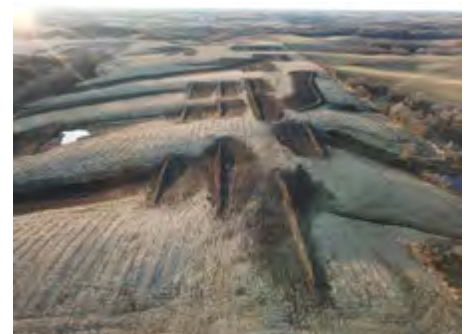
Newly constructed terraces in the Rathbun Lake Watershed in Southern Iowa
