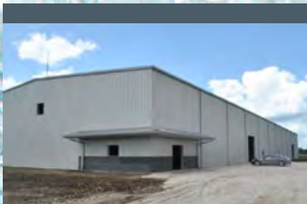
Fairfield Spec Exterior
