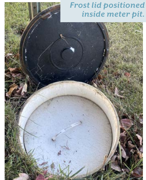
Properly placed lid on top of meter pit.
