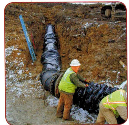
Installation of one of RRWA's new raw water transmission mains.
